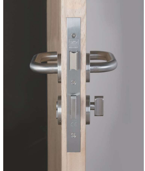
Figure 1 - Lock case fitted squarely within the door
